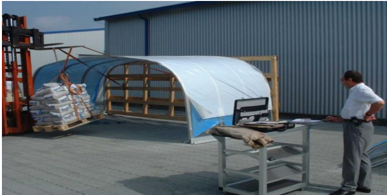
Test construction for the yearly check of German Technical Inspections Board (TUEV)
